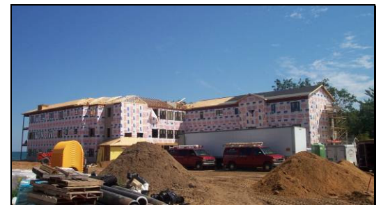
Building under construction
