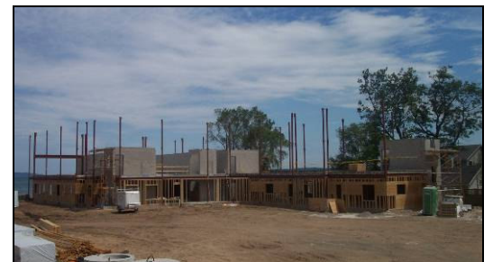
Building under construction
