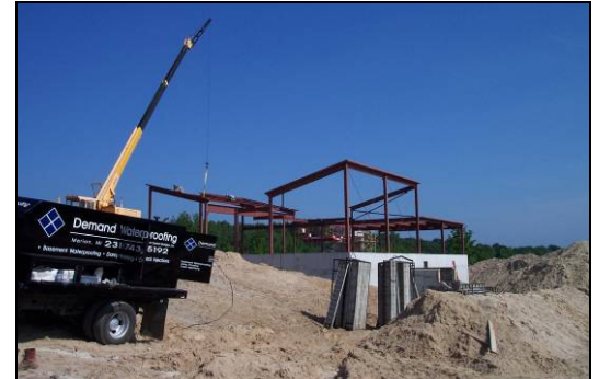
Building under construction
