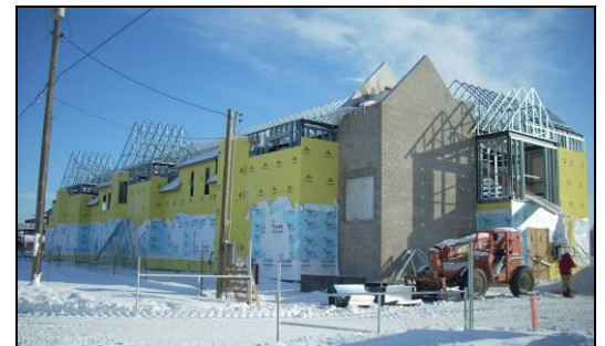
Building under construction
