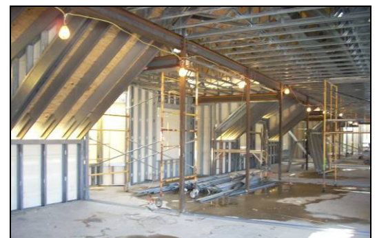
Building under construction
