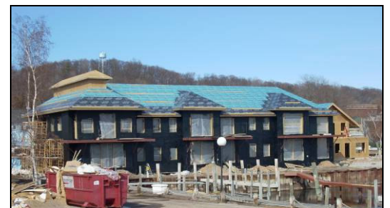
Building under construction
