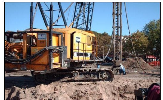
Installation of auger cast piling
