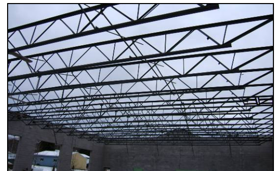
Building under construction
