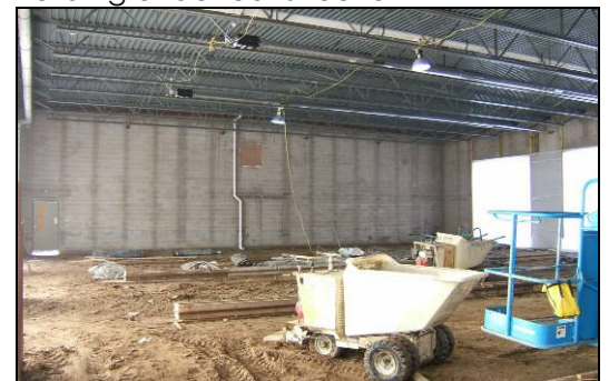
Building under construction
